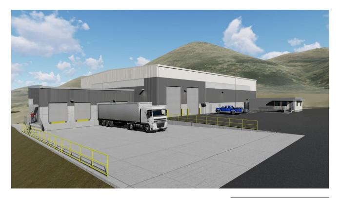
BREA, Calif. – JRMA (J.R. Miller & Associates, Inc.) is teamed with Golder Associates, Inc. to design a new transfer station building at the Tehachapi Landfill in Kern County, CA. The project includes a 300 ton per day (TPD) transfer station with a transfer tunnel for top loading, loading dock for recovered goods, public drop-off area, and a modular administration building.
